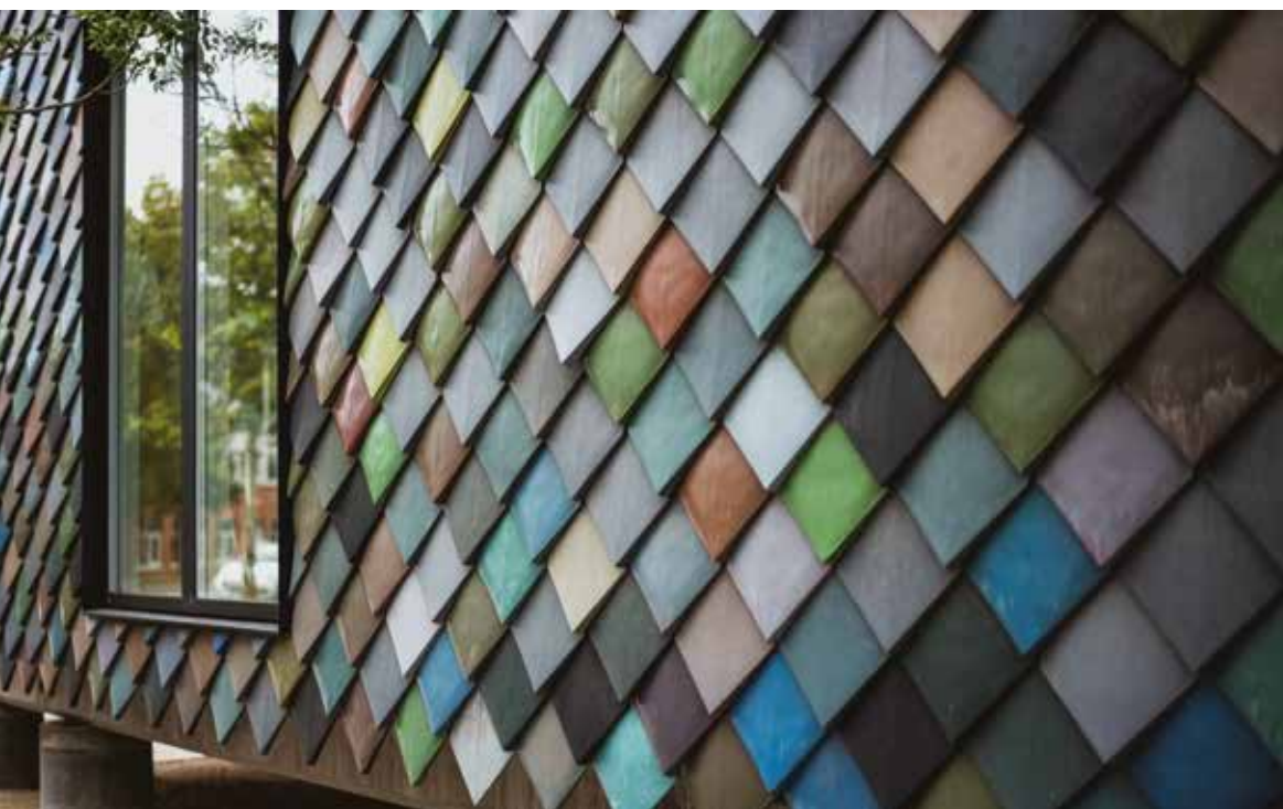
GEVEL VAN UPCYCLED PLASTIC (CIRCLE HOUSE, AARHUS).
